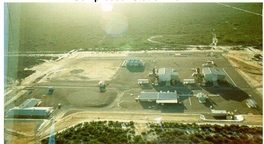
Compressor Station No 2
